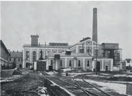
The company’s first production facilities were located in the former sugar factory premises in Čelechovice na Hané.
